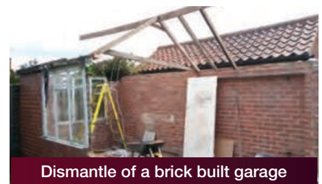
Old damaged roof being replaced
